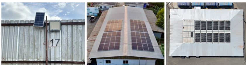
Figure: Solar Cell Installation
