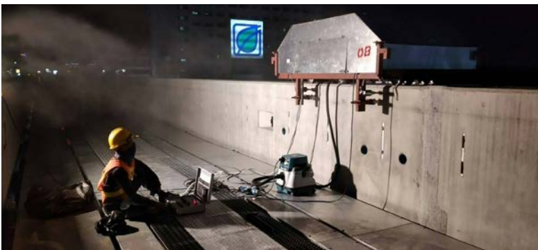
(Automatic GWB top grinding machine designed to flatten the upper surface of GWB wet joint connection)
