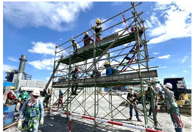
(Training in the “Scaffolding Installation Supervisor and Inspector” Course.)
