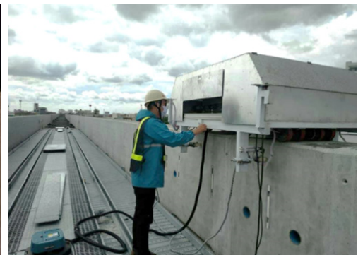
(Automatic GWB top grinding machine designed to flatten the upper surface of GWB wet joint connection)
